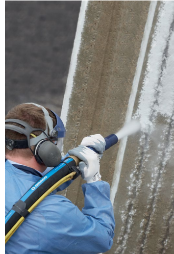
150 psi: Abrasive blasting
